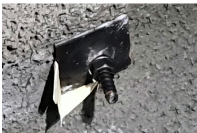
Figure 1. Post-injected resin gives clear evidence that rock bolt is fully encapsulated, and the two components (A + B) are perfectly mixed.
